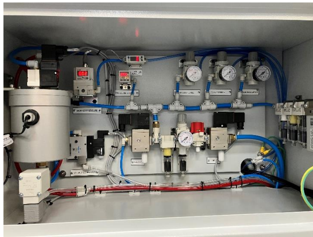
Figure 4 - Pneumatics / hydraulics cabinet
